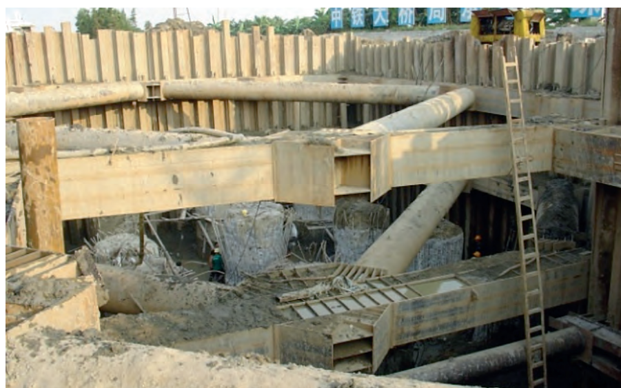
Fig. 13. Steel sheet pile cofferdam
