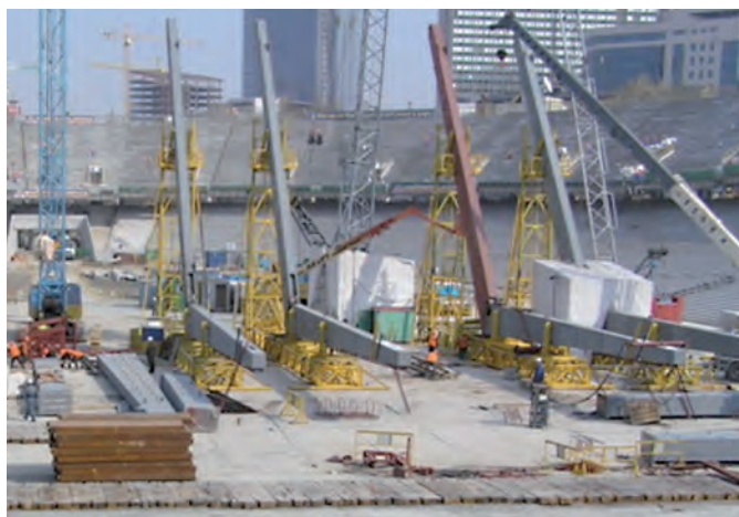
Fig. 6. A general view of the benches for assembling the column segments into larger sections on site
