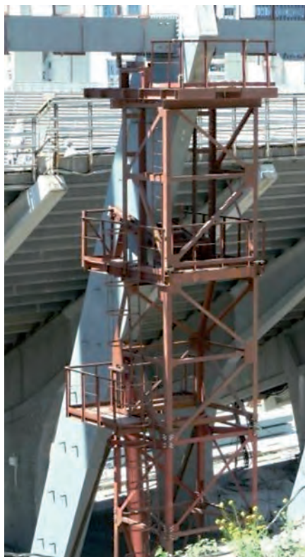
Fig. 7. A travelling tower for installing columns at their design positions and regulating their geometry
