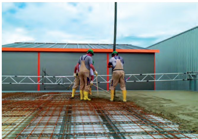
Fig. 1. Concreting the Cofraplus 220 floor system
