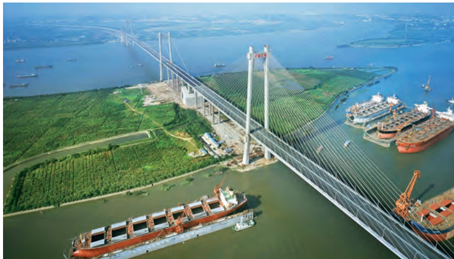
Fig. 15. The completed main bridge
