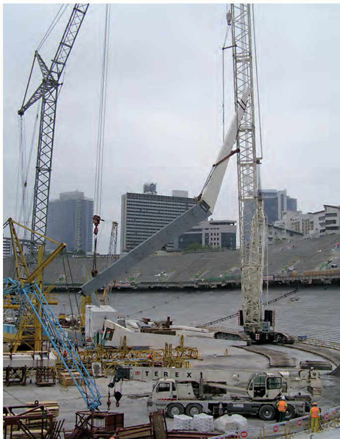
Fig. 9. Installing a column with the Demag CC 2800-1 and SKG-100 cranes
