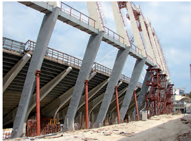
Fig. 8. Temporary props under the columns during erection
